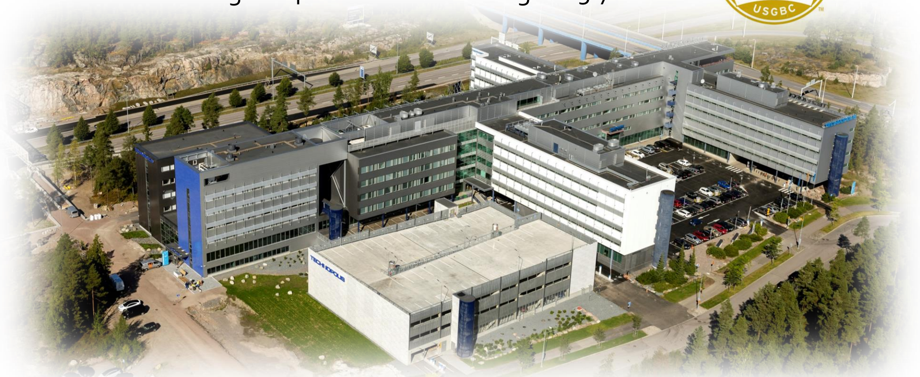
Vantaa campus with new G-building and parking garage
